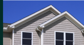
FASCIALS, SOFFITS & RAINWATER
