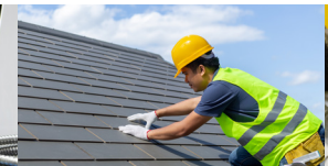
ROOFING & DRY VERGE
